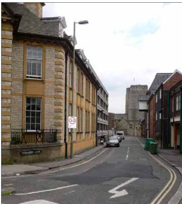
Tidmarsh Lane, the rear of Macclesfield House to the left, beyond the 1911-14 County Offices
